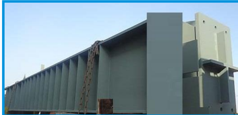
COLUMNS WITH BLASTING AND PAINTING
